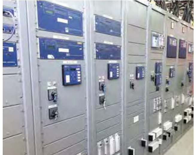
Some of the switchboard inside the upgraded Westmoorings Substation.
